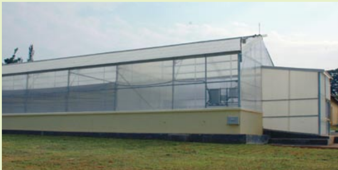
Exterior of the Containment Greenhouse
